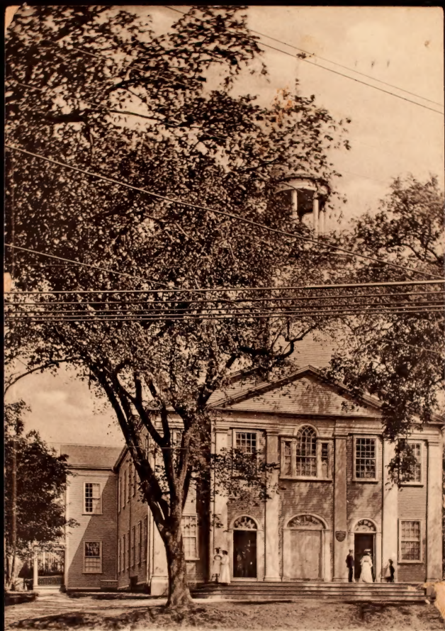
The New North. Gov. Long's Church. Hingham. Mass.
